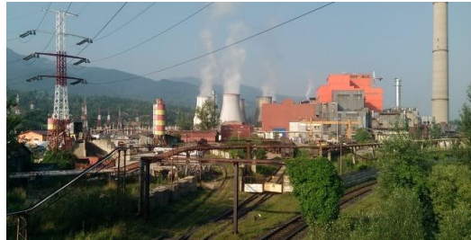
Figure 1 Paroseni Heating Power Plant
